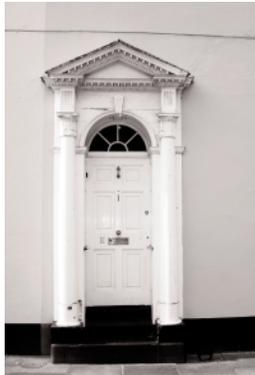
**Doors** would be pine and painted inside and out. (They would be made of 'pitch pine', a far superior wood to that which is available today.) You should always try to repair a door, but if it is not possible and you need to find more appropriate doors to replace uncharacteristic ones, try a salvage yard.
