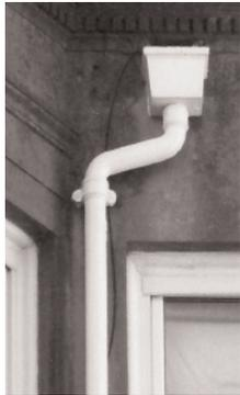
**Gutters** should be cast-iron. They are still made and are available through builders' merchants. They are heavy to replace, but are authentic and have a good life expectancy, unlike plastic, which can twist, expand and come apart at the joins.
