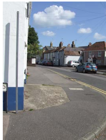
Pavement tarmacked in West Street
